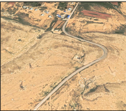
Fig Tree RAP on left near large bend
