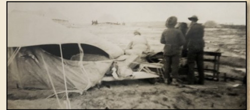
Tents flattened by tornado
